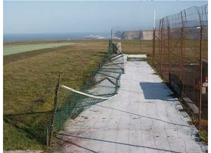
Our poor fence posts finally rusted through and the storm winds knocked our fence down. A temp fix has been made.
