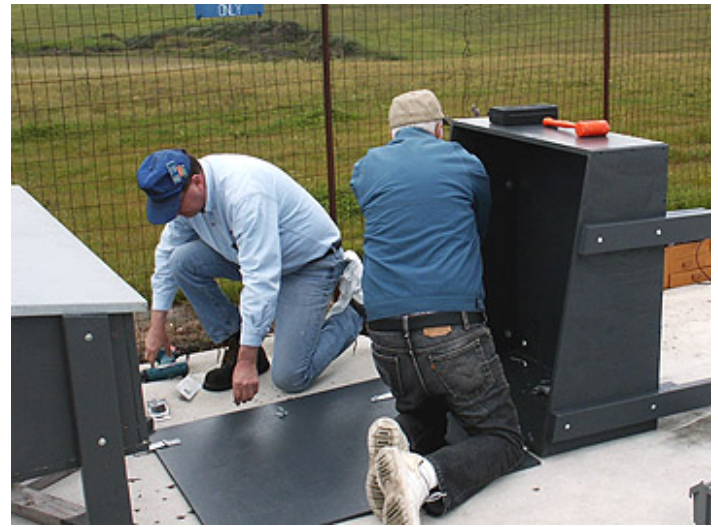
Dennis and Bob working on the new 'phone' box.
